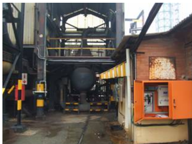
Photograph of the No. 9 Ammonia Oxidation Reactor structure and the analyser box
